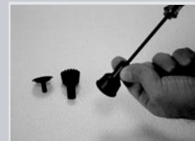
Clean the sprinkler head by using a screwdriver
